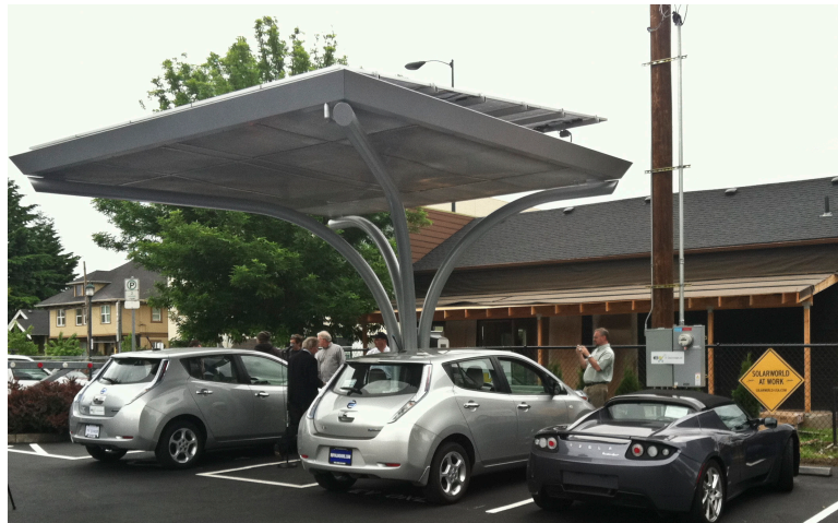
Figure 11: Solar canopy with EVSE at light rail station in Portland, Oregon (Source: Portland Development Corporation).
