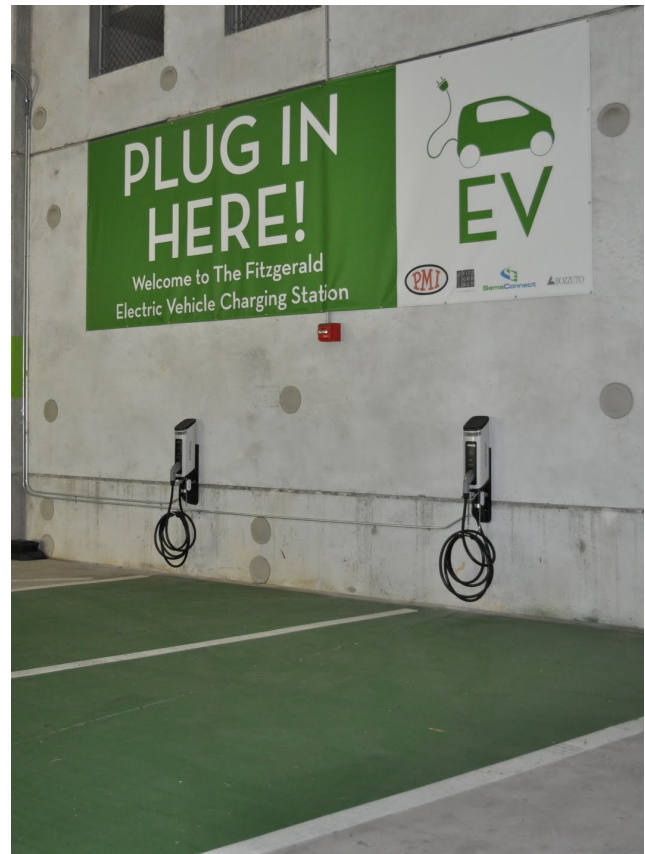
Figure 12: EVSE in the parking garage of The Fitzgerald, a 2011 multi-family development of the Bozzuto Group. (Source: SemaConnect http://semaconnect.blogspot.com/2011/06/charging-landscape.html ).
