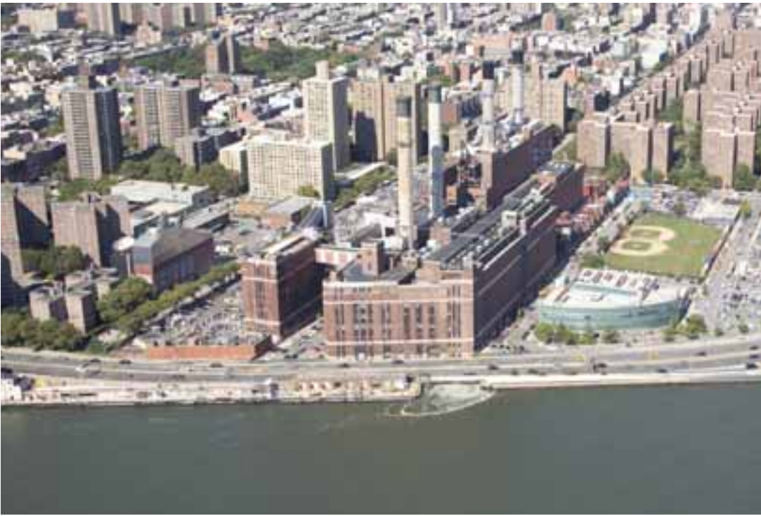
Bird's-eye view of existing pinch point looking west
