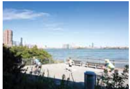
Existing bulkhead at Stuyvesant Cove
