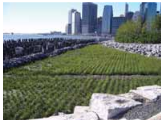
Salt marsh and construction and pier removal at Brooklyn Bridge Park
