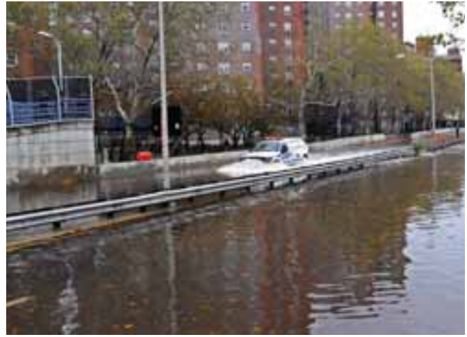
Flooding on the FDR Drive after Hurricane Sandy
