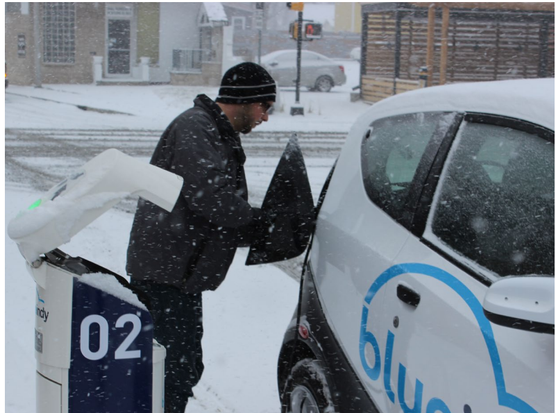
Figure 39: Single-port charging stations installed curbside in Indianapolis, Indiana. (Image courtesy of BlueIndy)
