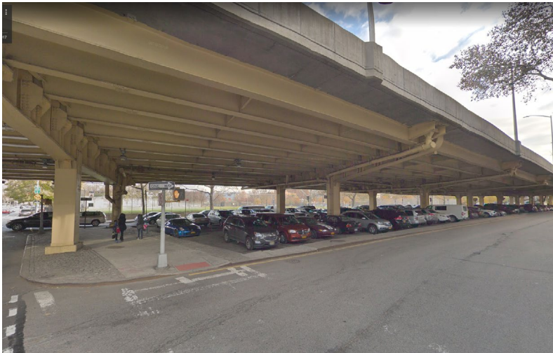
Figure 23: Front-in parking under the Brooklyn-Queens Expressway, Park Avenue at Navy Street, Brooklyn (Streetview ©2018 Google)
