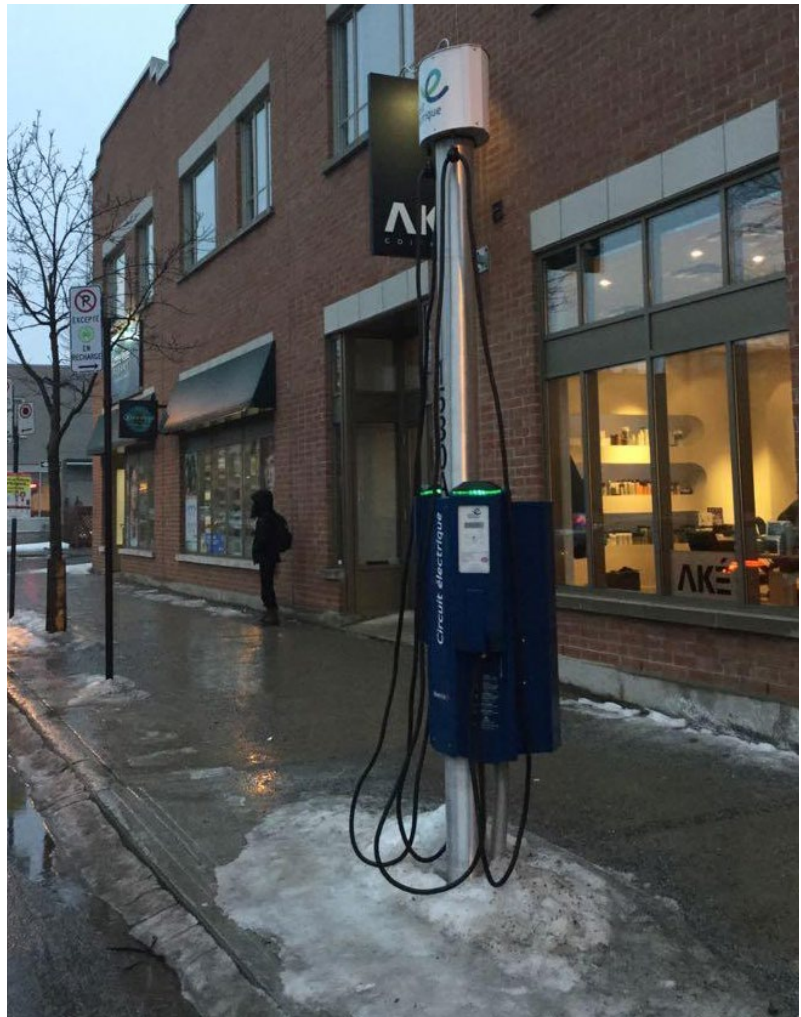
Figure 38: Dual-port curbside installation in Montréal, Canada, where harsh winter weather requires a durable charging solution. (Image courtesy of Flo)
