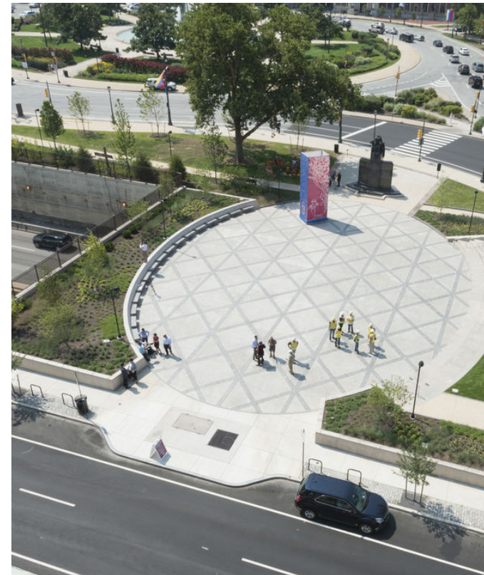
Partial trench cover
