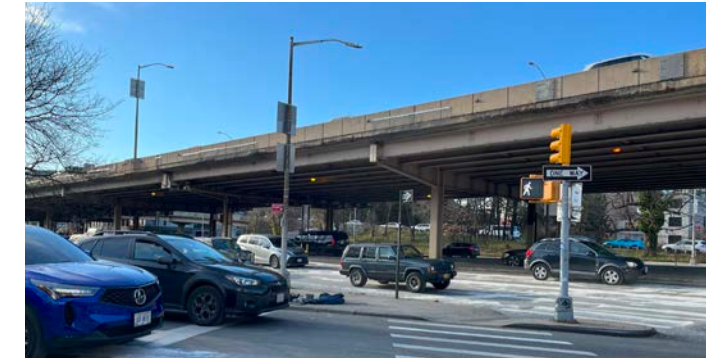
Meeker Ave. and Humboldt St.
