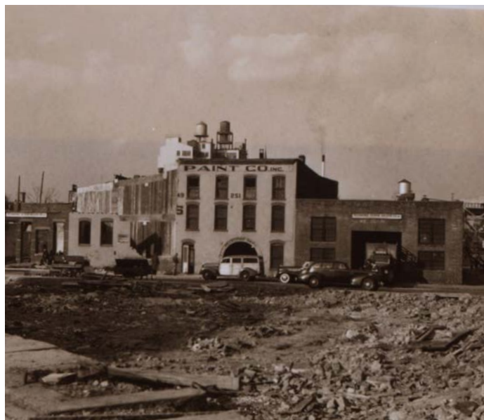
2 Hamilton Ave. and Smith St., before (1940) the BQE.
