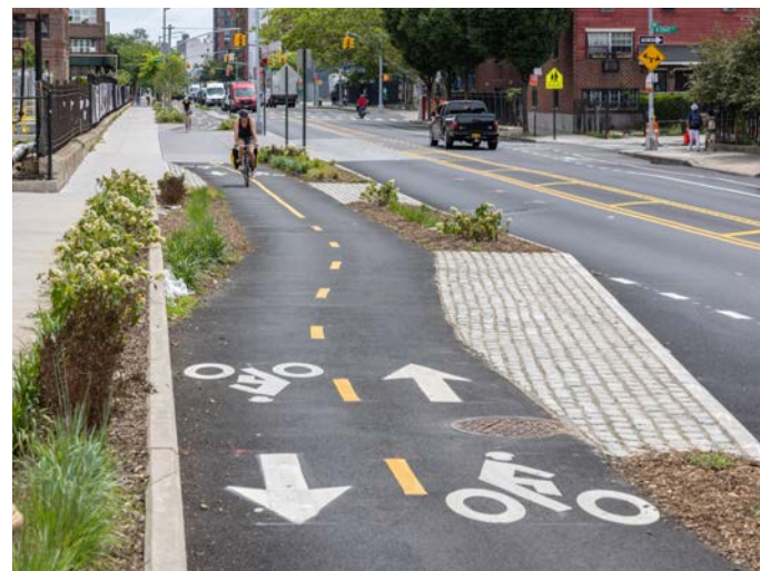
Grade-separated bike lane
