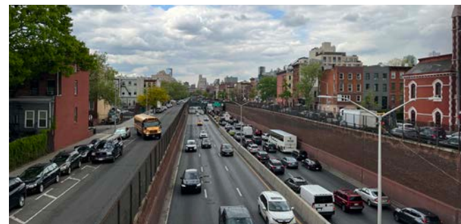
BQE trench view from bridge
