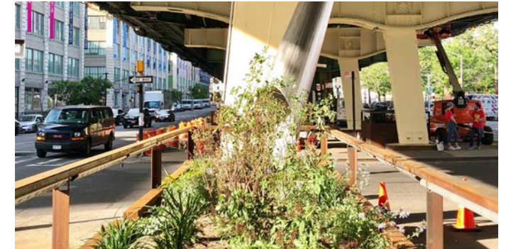
Cone-like downspouts capture storm water from the BQE elevated structures (EI-Space Pilot in Sunset Park, Brooklyn)
