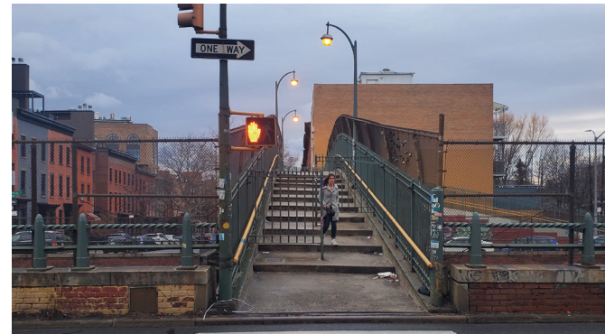
Existing Summit St. pedestrian bridge
