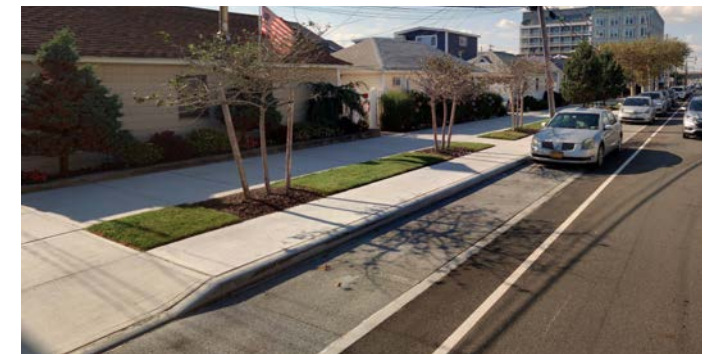
Porous concrete in the parking lane on Beach 108th St. (Rockaway Beach, Queens)
