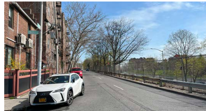
90th St. and Gatling Pl. looking north over the BQE
