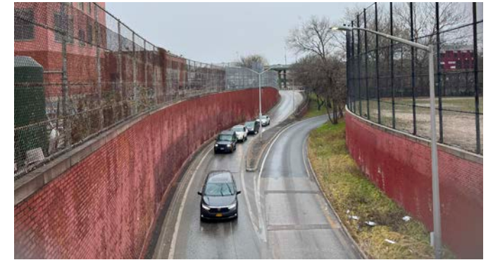
On-ramp at Rapelye St./Exit 26
