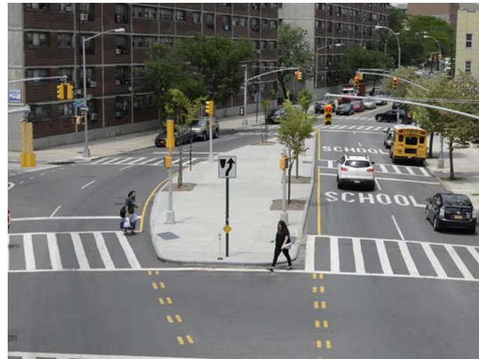
Concrete median and curb extensions
