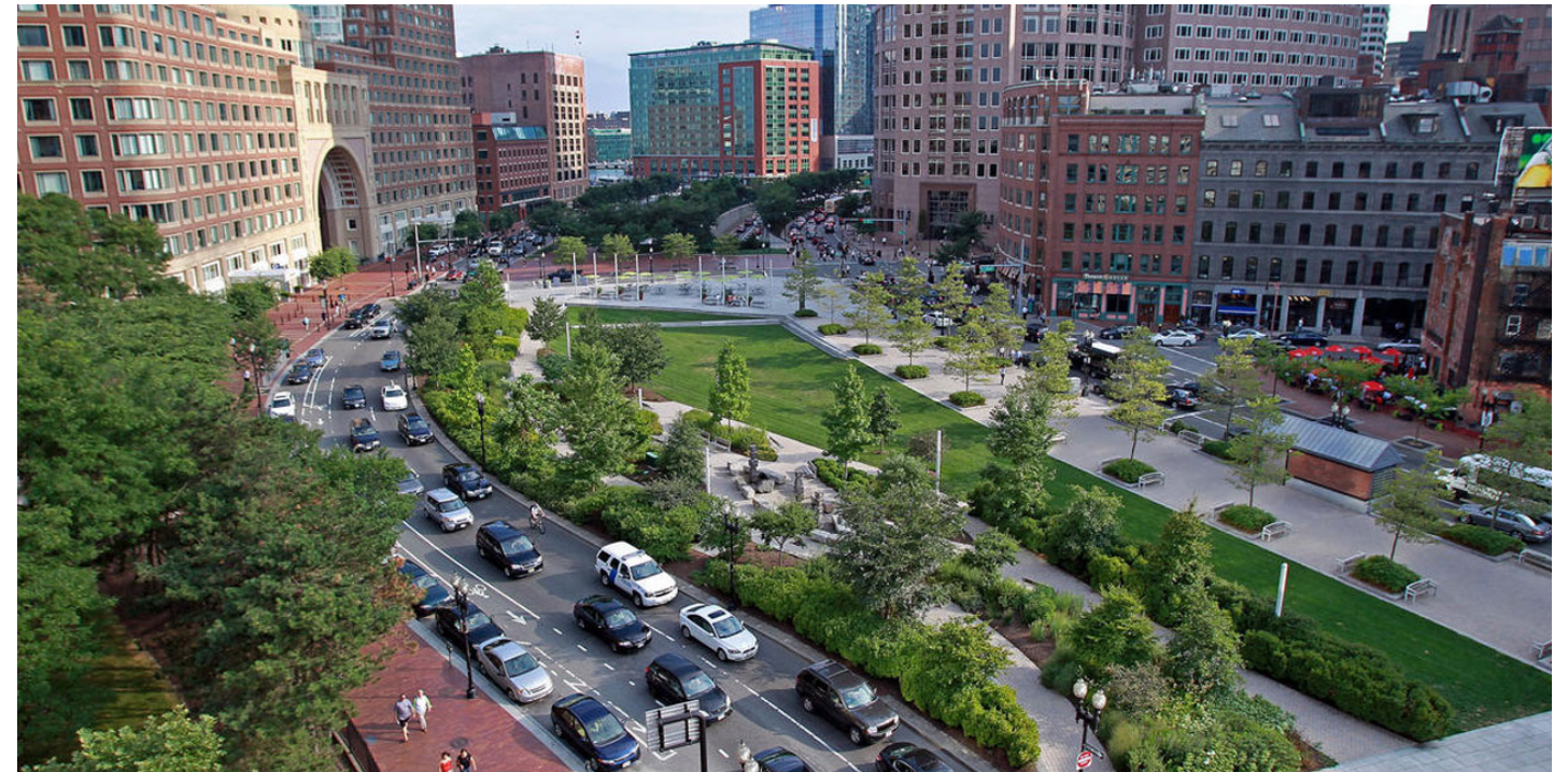
Highway tunnel with open space (Boston, MA)
