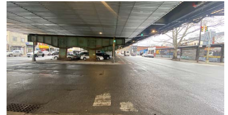
Third Ave. elevated structure
