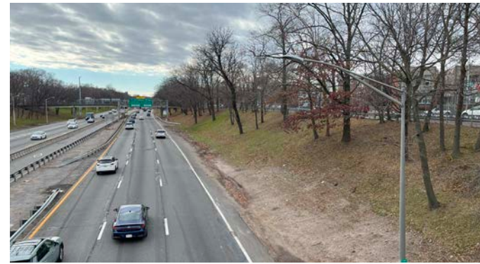
Bay Ridge Pkwy. bridge looking north over the BQE
