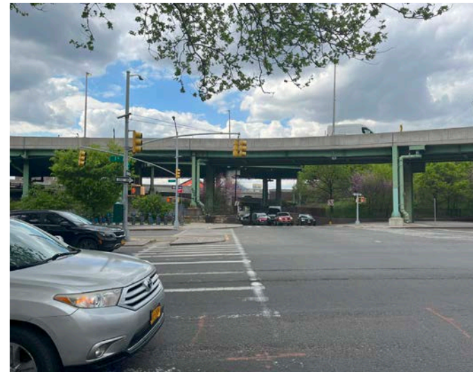
Existing pedestrian crossing at 17th St. and Third Ave.
