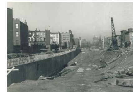
Cobble Hill trench under construction 1950s
