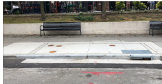
Concrete top infiltration basin
