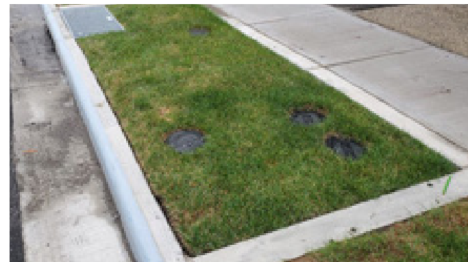
Grass top infiltration basin
