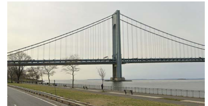
Shore Pkwy. looking south towards Bay Ridge Promenade
