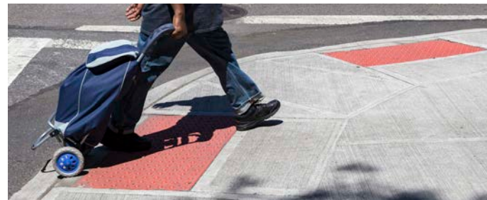
Pedestrian walking across textured ramp
