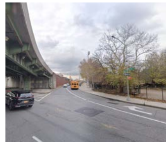
2 Hamilton Ave. and Hicks St., before (1931) and after (2023) the BQE.
