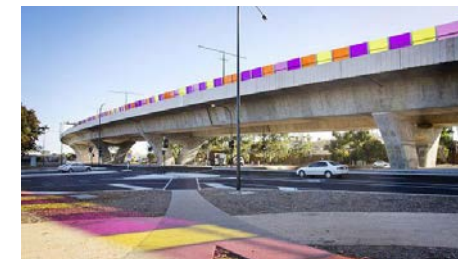
Acoustic barrier (Adelaide, Australia)
