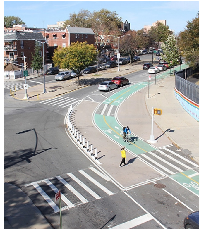
Protected bike and pedestrian barrier at 111th St. and Corona Ave. (Queens, NY)
