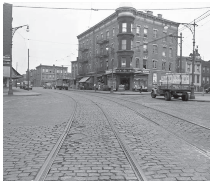
2 View from Richardson St. and Graham Ave. trolley line (#16), before (1944) the BQE.
