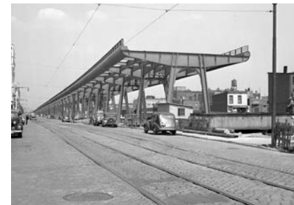
Third Ave. Elevated, 1941
