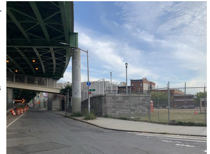
View of existing Red Hook Footbridge from Hamilton Ave.
