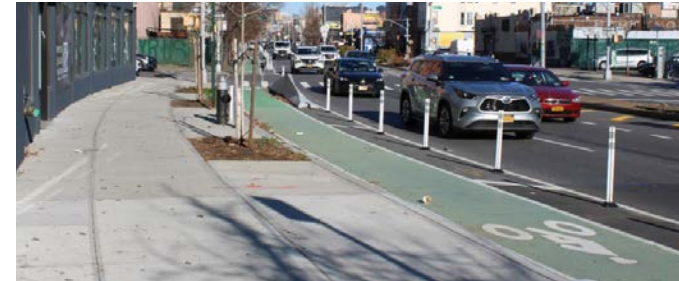
New bike lane on McGuinness Blvd.
