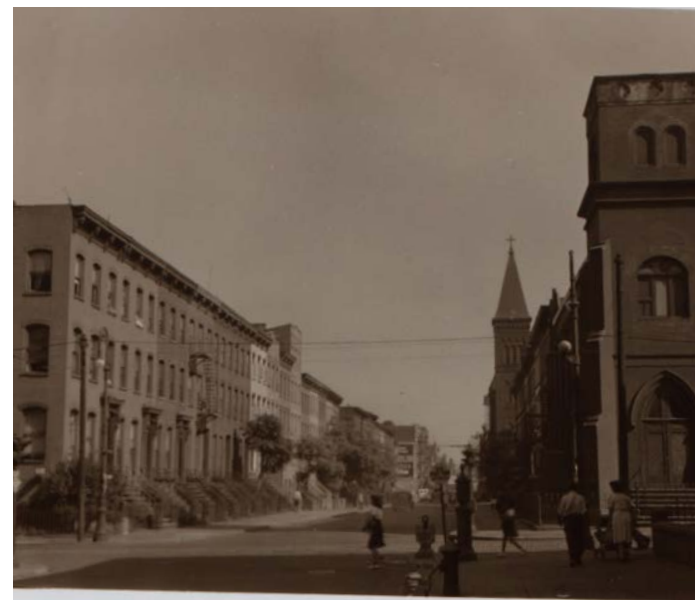
3 View from S 5th St. and Marcy Ave, before (1941) the BQE.
