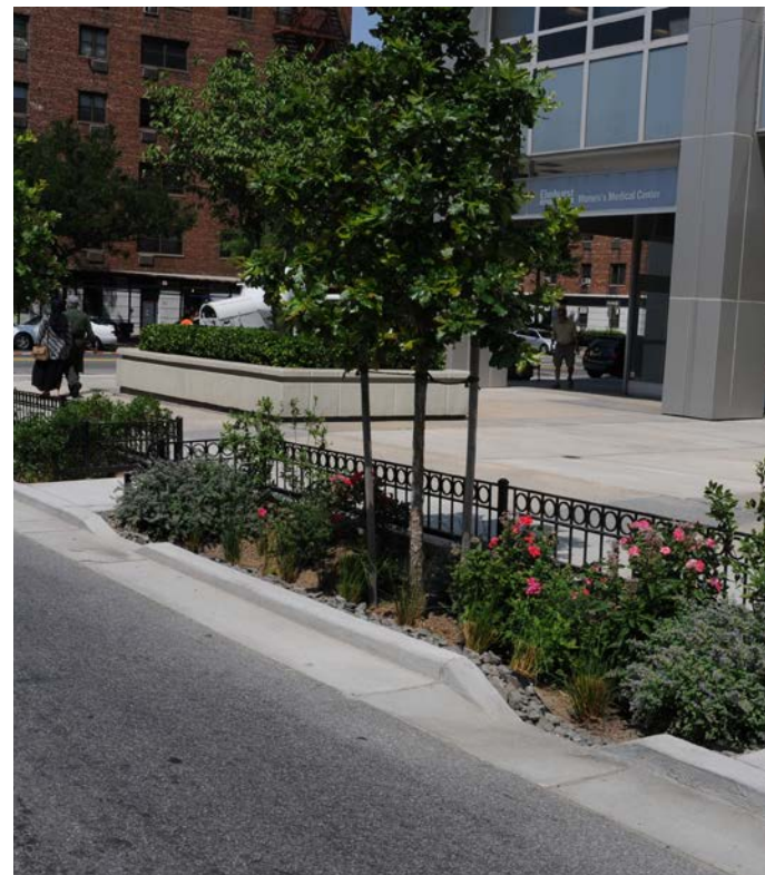
Rain gardens (Elmhurst, Queens)
